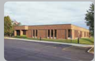
Headquarters Willowbrook, Illinois.
